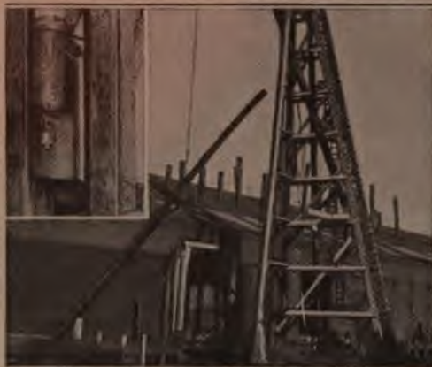
When the Boom is Not in Use, It is Tied Fast to the Pile Driver, in Such a Manner That It Does Not Interfere with the Operation of the Hammer
